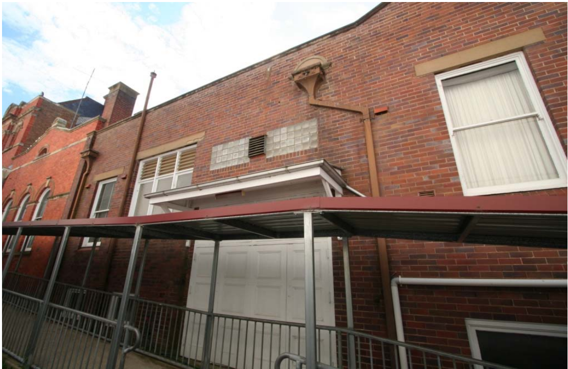
Photograph 14 A detail view of the South Elevation noting the junction between the original the addition with the replacement Town Hall
