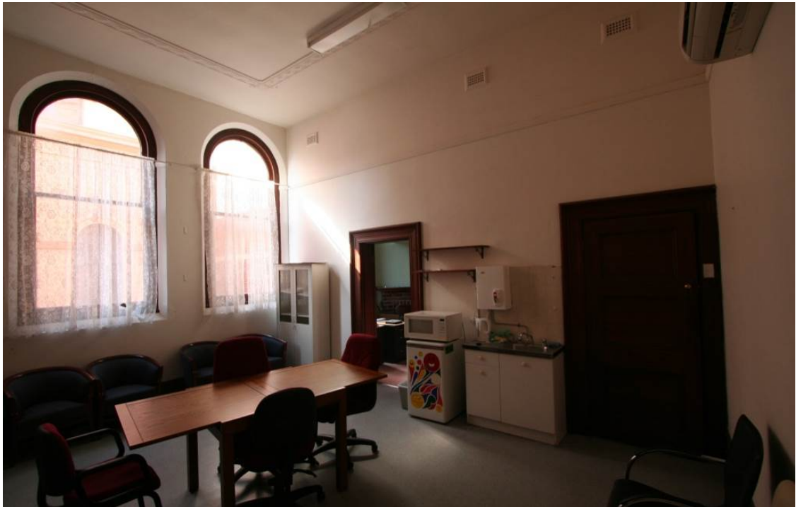
Photograph 24 Wall and joinery formed for the later Town Hall to be demolished and the vaulted ceiling reinstated.
